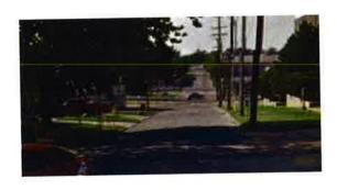
lanes flanking 10-foot lanes. (Street Type 36-BDDB). The short segment between 1<sup>st</sup> Street and Heavy Traffic Way is even wider: a 44-foot cartpath holding two driving lanes. Here, in addition to the provision of bike lanes, a parallel parking lane should be added against the west curb. (Street Type 44-PBDDB)
